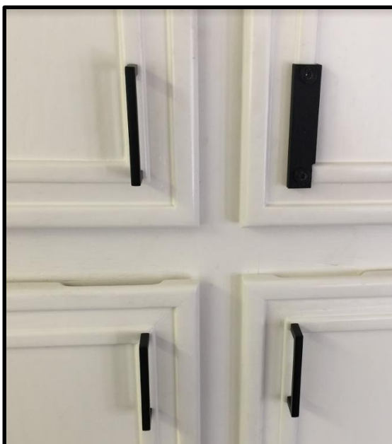
Holes drilled and new hardware successfully installed
