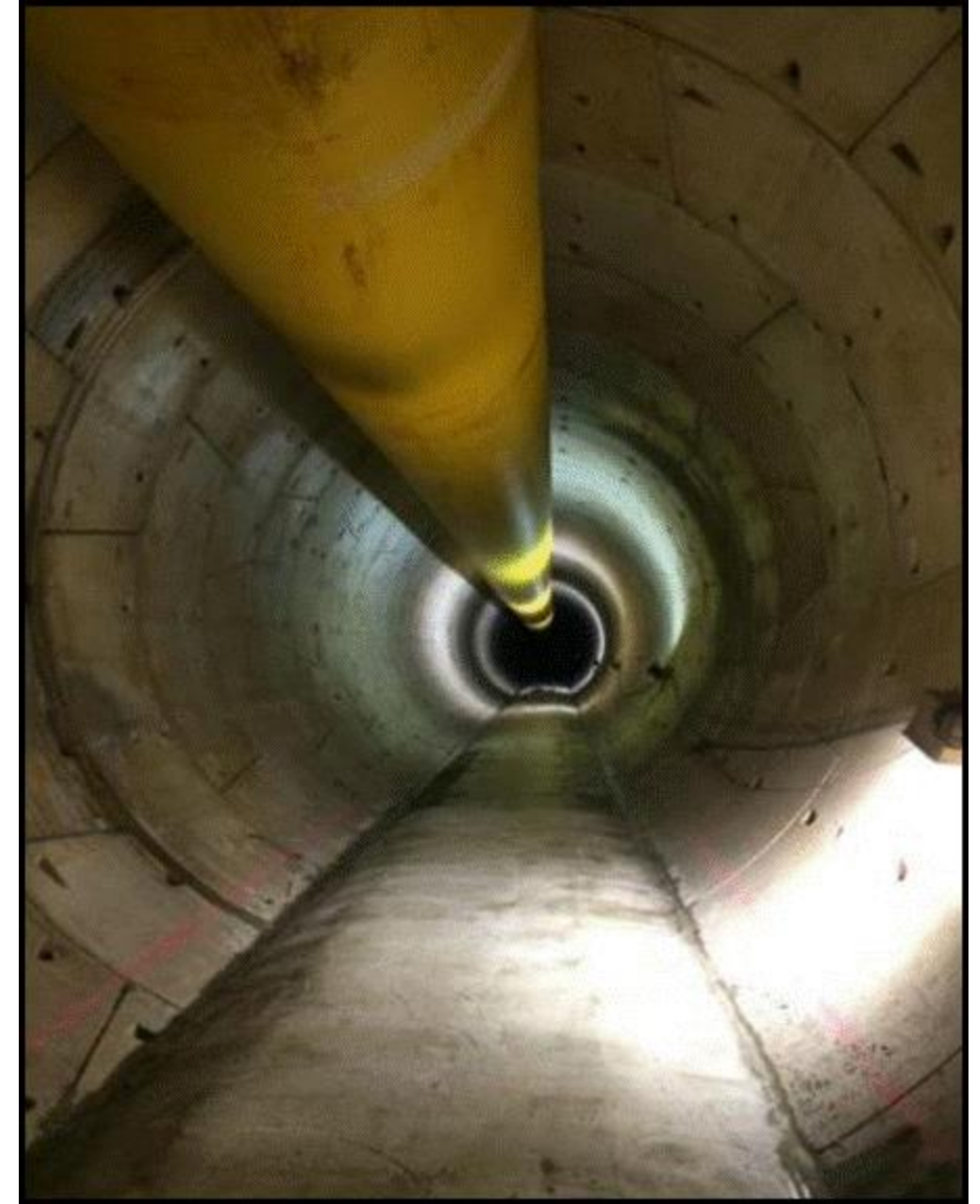
Before Intake No. 3 was put into service
